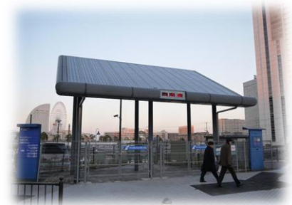
Figure 1: Solar-assisted clock in Yokohama
